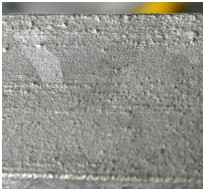
Fig 1. Uneven coating due to variable surface steel chemistry
